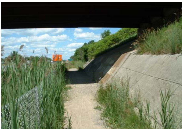
The Cherry Hill Viaduct
